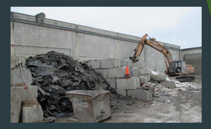
Asphalt Shingles, Sheet Rock, and other Inert Debris Bunkers
