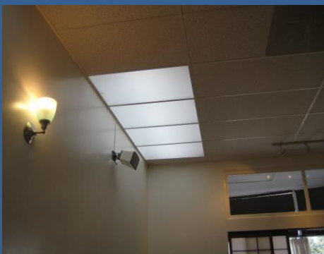
Fluorescent lamps in the "skylight" at left mimic the natural daylight spectrum, while the clerestory window at right lets natural light from the reception area reach the studio.
