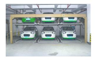
readily to reuse and recycling. The structures housing the systems can also be better designed for future adaptive reuse than conventional structures. CityLift's Hive parking structure in Oakland is the first fully automated parking structure in the Bay Area and houses 39 spaces in the footprint of seven surface-level spaces, or 1,600 square feet.
