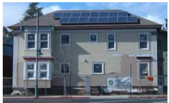
Magnolia Terrace under construction, March 2011
