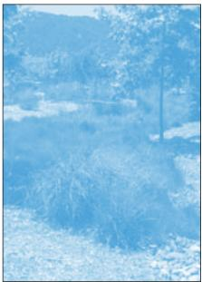
Site water flows to a bioswale, enhancing on-site infiltration and reducing contaminants.
