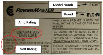
Figure 13. Example of a Subpanel Nameplate
