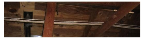
Figure 15. Feeder Cables in an Attic
