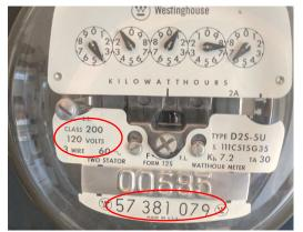
Figure 19. Meter Showing Voltage and Meter Number
