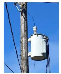
Figure 23. Pole-Mounted Transformer
