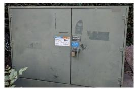
Figure 24. Pad-Mounted Transformer
