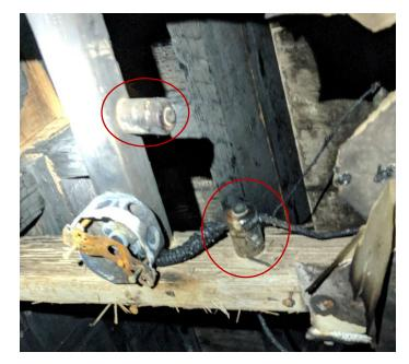
Figure 17. Knob and Tube Wiring
