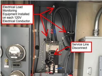
Figure 26. Load Monitoring Equipment
