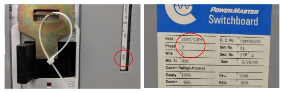
Figure 20. Service Disconnect and Switchboard of a Large Multifamily Building
