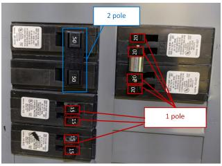
Figure 11. Panel Showing Single- and Dual-Pole Breakers
