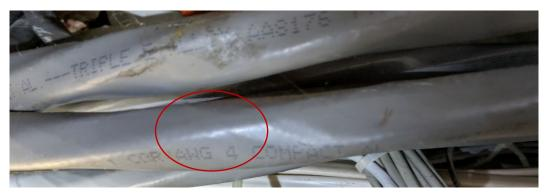
Figure 16. AWG Rating Visible on Exposed Feeder Cables
