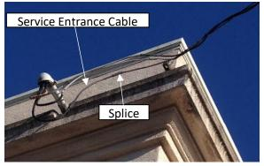
**Figure 22. Service Drop Spliced to Service Entrance Cables**
