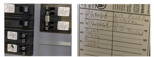
Figure 10. Subpanel Labeling
