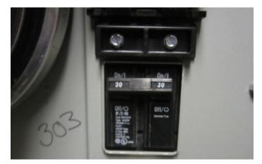
Figure 18. 30 A Dual-Pole Secondary Disconnect Next to a Meter
